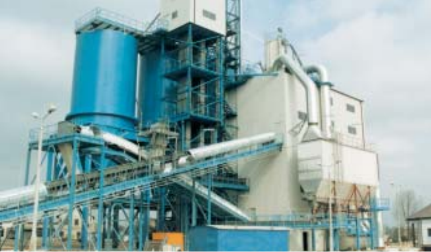
The new grinding plant at Wolica, Poland, was opened in June 2001.
